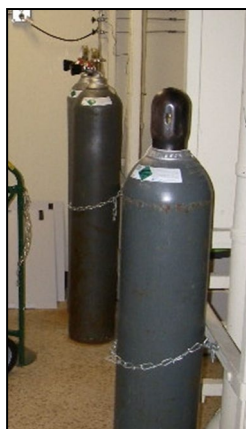
Acceptable method of securing a gas cylinder
