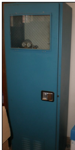
Compressed gas cylinder cabinet
