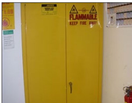
Proper storage of flammable chemicals
