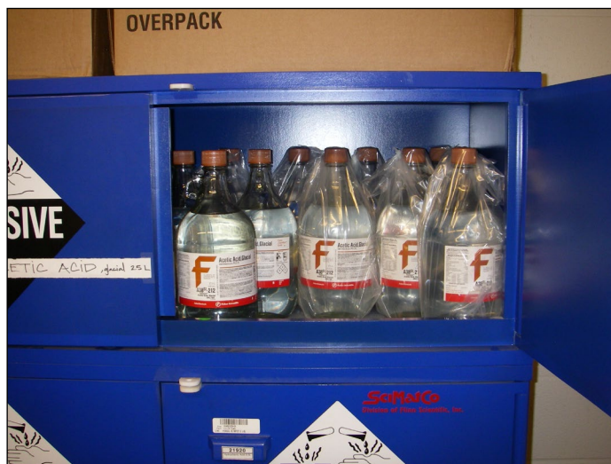
Acids stored in acid storage cabinet
