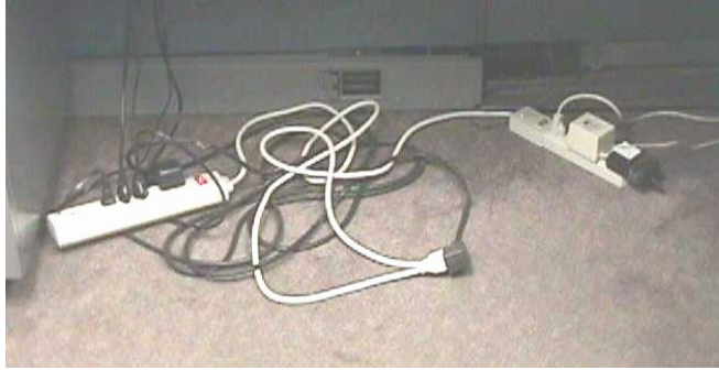
Overloaded multi-plug strip
