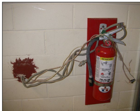
Blocked fire extinguisher
